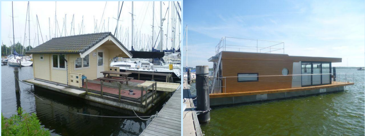
Example for a floating cabin in Muiderzand (left) aiming to attract e.g. family members of resident boaters and freely accessible for those, and a floating house in Kröslin (right) both swimming in a berth, freely manoeuvrable and officially not counting as house as they are too small and built on a ship body.
