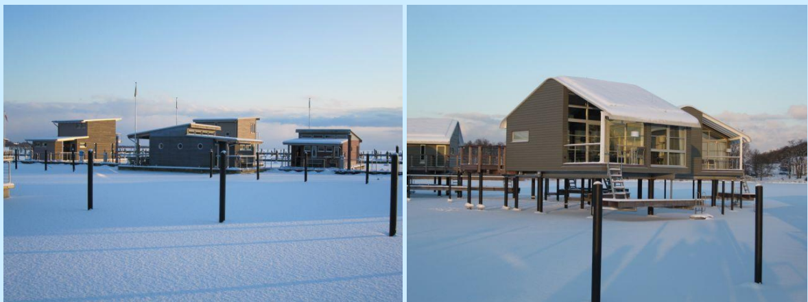
Example for bigger floating houses (left) in Lauterbach that need a building permission and a pile house (right) inspired by houses on the Seychelles.
